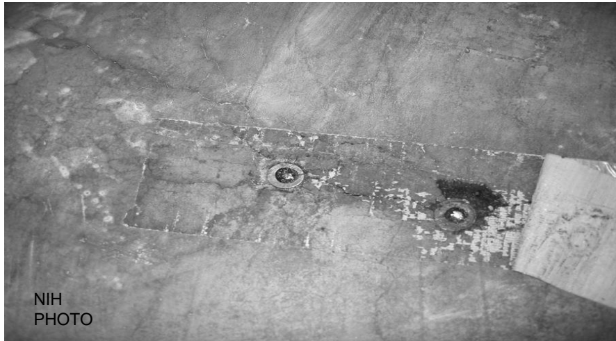
Mercury in expansion anchors found under vinyl asbestos tile
