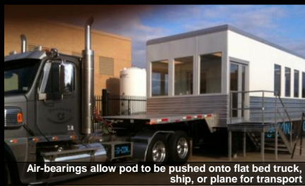
Requires only electrical hook-up and chilled water
